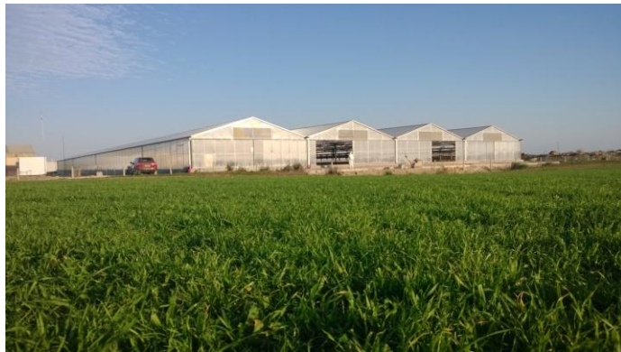
Exterior view of the plant
