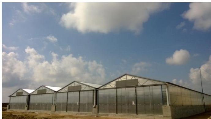
Exterior view of the plant
